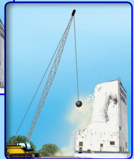
A wrecking ball on a short chain (above) cannot be lifted as high and hits the wall with less energy than a wrecking ball on a longer chain (right).
